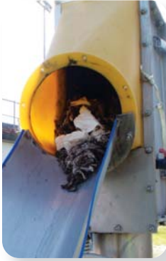
Discharge spout using SINT® Techno-polymeric material.
