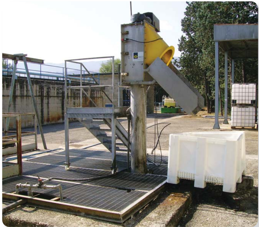
Open Channel Installation
